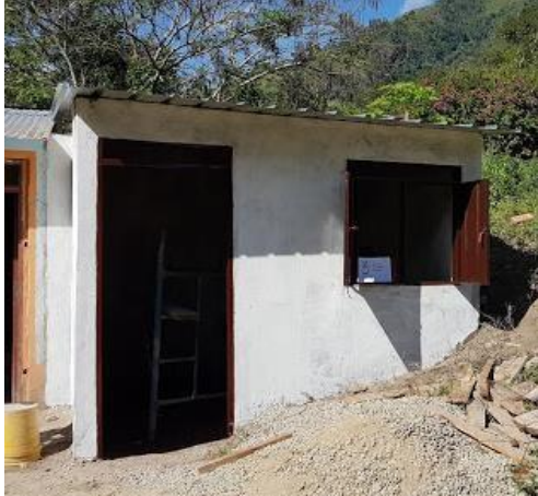
Foto No. 5: fachada principal
